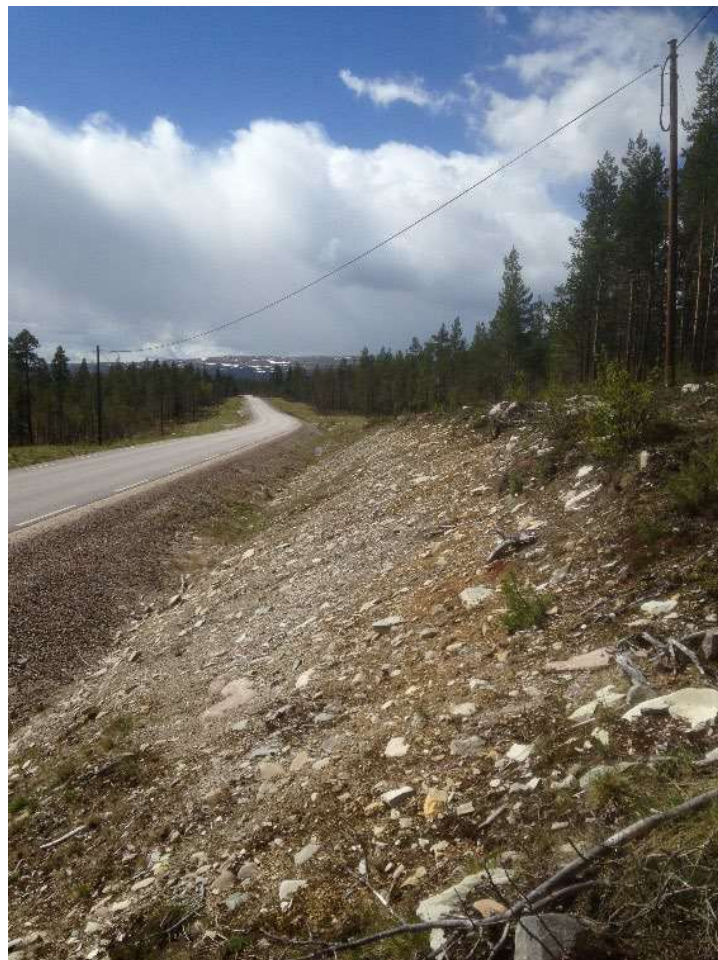
Figure 2.1.3-1: Re-use of topsoil to restore road verges after road rehabilitation approx. 600 m.a.s.l., Fylkesveg 2208 Engerdal municipality, Innlandet county. Photo: Line Rosef
