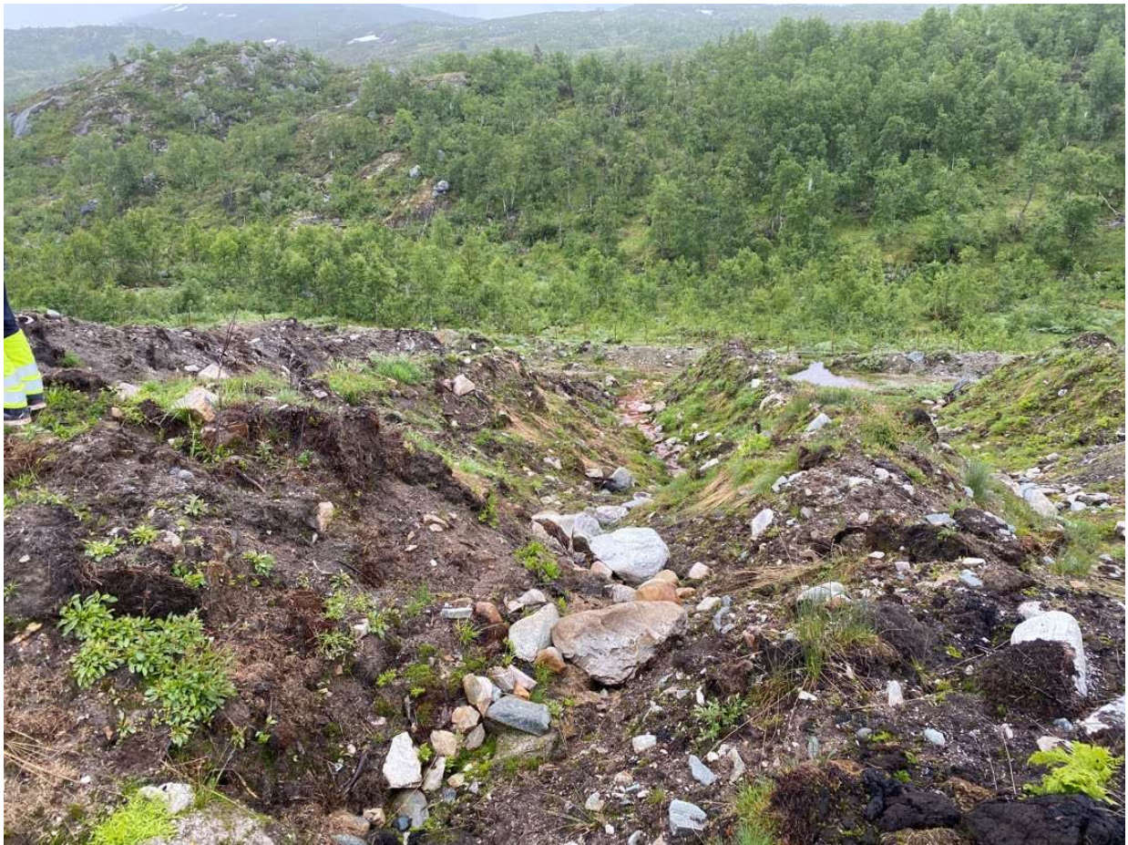
Figure 2.3.2-1: Soil heaps of organic topsoil, approx. 960 m.a.s.l., Songa dam, Vinje municipality, Vestfold and Telemark County. Photo: Line Rosef
