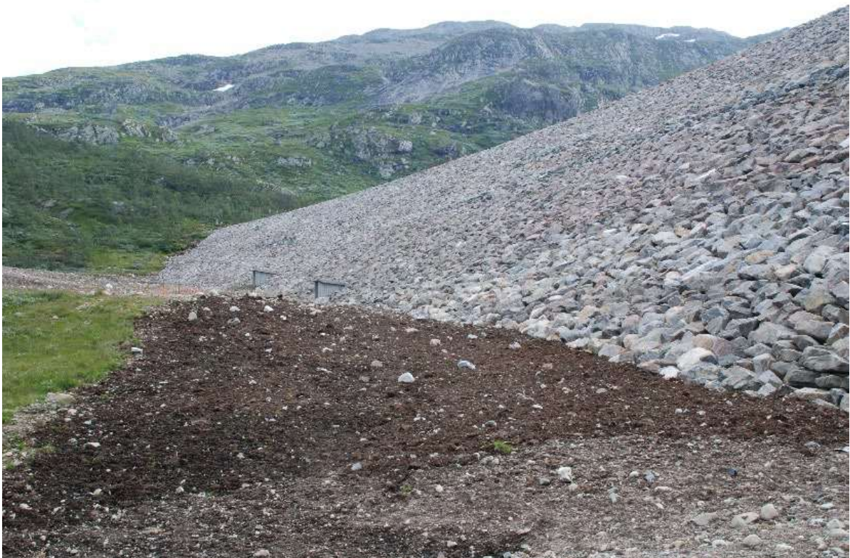
Figure 2.1.5-1: Restoration of landscape and vegetation after hydroelectric power dam rehabilitation approx. 950 m.a.s.l., Bitdalen dam, Vinje municipality, Vestfold and Telemark County. Photo: Line Rosef
