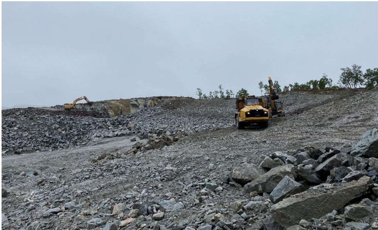
Figure 2.1.5-2: Stone quarry for hydroelectric power dam rehabilitation approx. 960 m.a.s.l., Songa dam, Vinje municipality, Vestfold and Telemark County. Photo: Line Rosef
