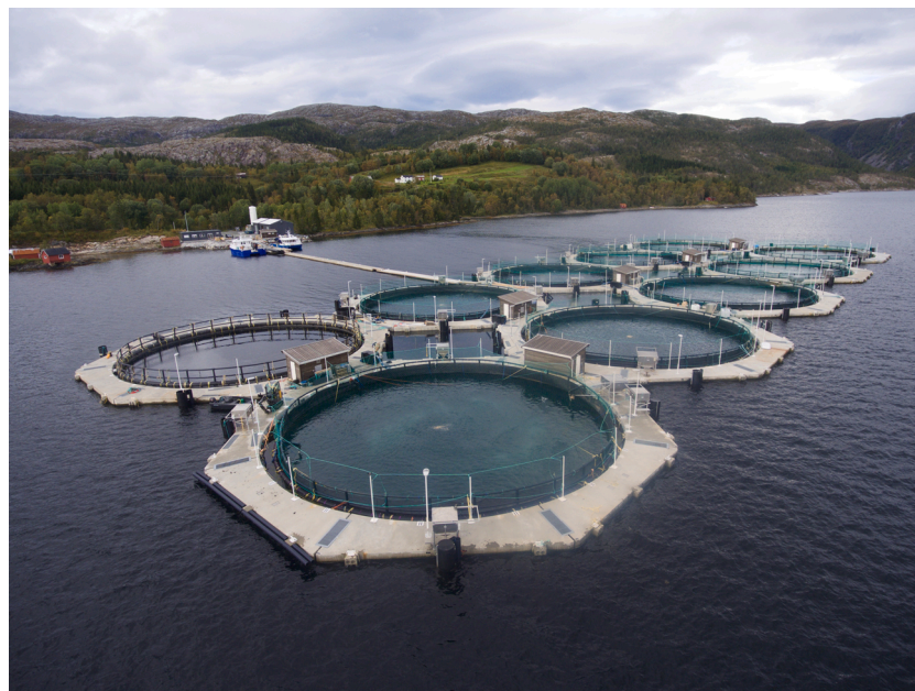
Fig. 3. Site 3 with 10 CCS, each with a volume of 6000 m 3 (Photo: AkvaFuture AS).
